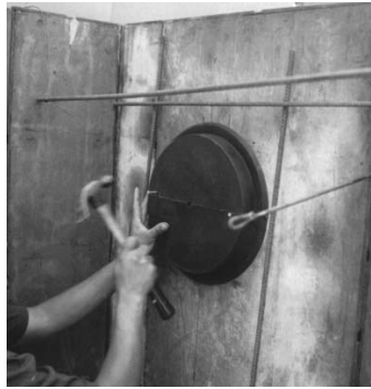
2. Nail one of the end caps at the marked center line. A 2" minimum clearance is suggested when nesting sleeves.
