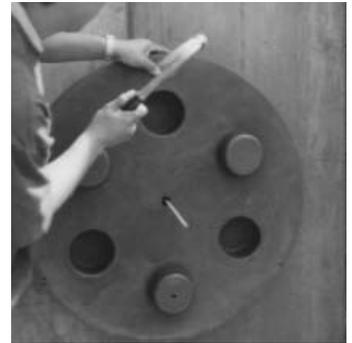
4. Secure the edges of the cell to the form using the provided steel spikes.
