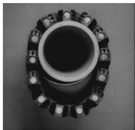
3. Check to be sure all bolt heads are facing the installer. Extra slack or sag is normal. Do not remove links if extra slack exists. **Note:** On smaller diameter pipe, links may need to be stretched.
