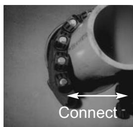
2. Loosen rear pressure plate with nut just enough so links move freely. Connect both ends of belt around the pipe.
