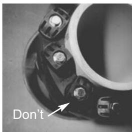
1. Don't Install the belt with the pressure plates aimed in irregular directions. (Staggered)
