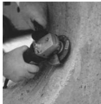
11. Inspect the installation. A smooth opening is important for a proper Link-Seal® modular seal installation. Repair voids and grind smooth any ridges.
