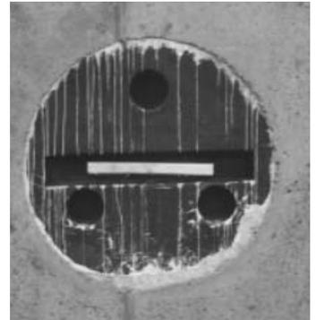
8. After wall cures, wall forms are removed. The Cell-Cast® disk assembly is now ready for removal.
