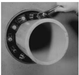
5a. **LS-325 thru. LS-650** Using a hand socket or off-set wrench **ONLY**, start at 12 O' Clock. Do not tighten any bolt more than 4 turns at a time. Continue in a clockwise manner until links have been uniformly compressed. (Approx. 2 or 3 rotations)
