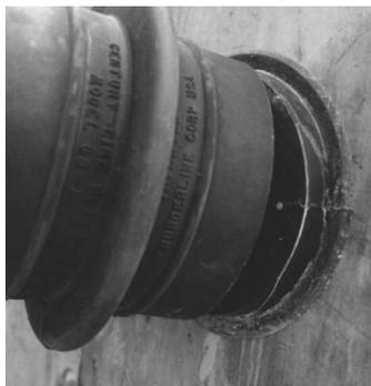
3. Place the Century-Line® Sleeve on the end cap. *When field cutting non standard CS sleeve lengths, the sleeve and endcaps total length should be one-fourth (1/4") longer than the thickness of the wall. Cut with a hand or power saw. Note: To insure minimum water migration, center the water stop in wall by cutting equal lengths from each end of the sleeve, as noted below.*
