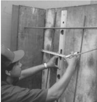
1. Measure the center line to position Century-Line® Sleeve end cap.
