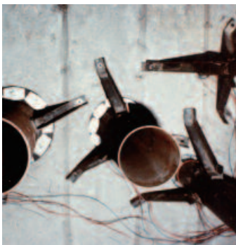
Certified test furnace with pipe and cable penetrations and fire rated Link-Seal® modular seal installed in concrete floor slab. Twenty-seven thermo couples were used per slab.
