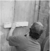
2. A 2x4 wood nailer is included. Fasten it along with the threaded rod directly to the concrete form. This provides support and helps center the complete Cell-Cast<sup>®</sup> disk assembly.
