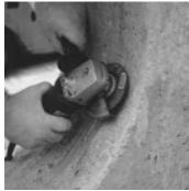
**11.** Inspect the installation. A smooth opening is important for a proper Link-Seal<sup>®</sup> modular seal installation. Repair voids and grind smooth any ridges.
