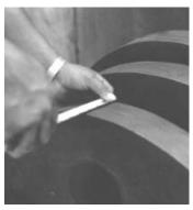
**5.** Additional disks are interlocked to accommodate finished wall thickness. Verify thickness is the same as wall.
