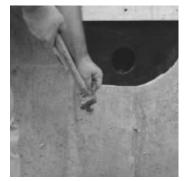
**9.** Chip excess concrete from the edge of the Cell-Cast<sup>®</sup> disk assembly and wall.
