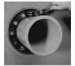
**5a. LS-325 thru. LS-650** Using a hand socket or off-set wrench ONLY, start at 12 O' Clock. Do not tighten any bolt more than 4 turns at a time. Continue in a clockwise manner until links have been uniformly compressed. (Approx. 2 or 3 rotations)
