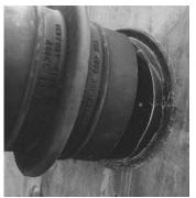
3. Place the Century-Line® Sleeve on the end cap. When field cutting non standard CS sleeve lengths, the sleeve and endcaps total length should be one-fourth (1/4") longer than the thickness of the wall. Cut with a hand or power saw. Note: To insure minimum water migration, center the water stop in wall by cutting equal lengths from each end of the sleeve, except as noted below.
