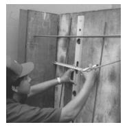
**1.** Measure the center line to position Century-Line<sup>®</sup> Sleeve end cap.
