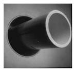
1. Center the pipe, cable or conduit in wall opening or casing. Make sure the pipe will be adequately supported on both ends. Link-Seal<sup>®</sup> modular seals are <u>not</u> intended to support the weight of the pipe.
