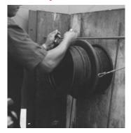
5. For additional stability, it's necessary to secure the sleeve with wire to the rebar. Insert the other end cap firmly, check that second end cap is positioned correctly, confirm sleeve length and close the form.
